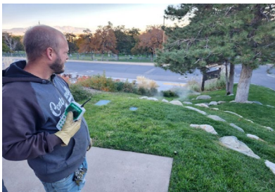
Parks employee, Tyler West, blows out sprinkler pipes in the fall.
